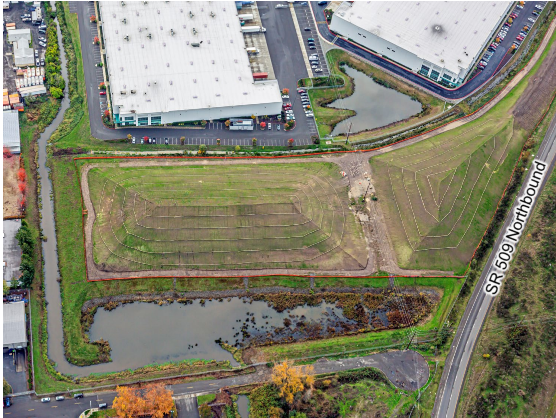
WSDOT Stockpiles (~180,000 CY)
